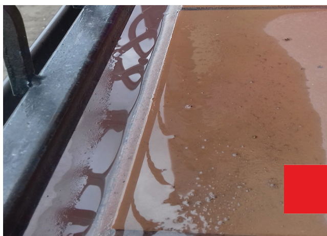
IMPROPER DRAINING OF WATER FROM THE FLOORING
