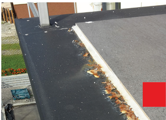
DRIP TRAYS CORROSION
